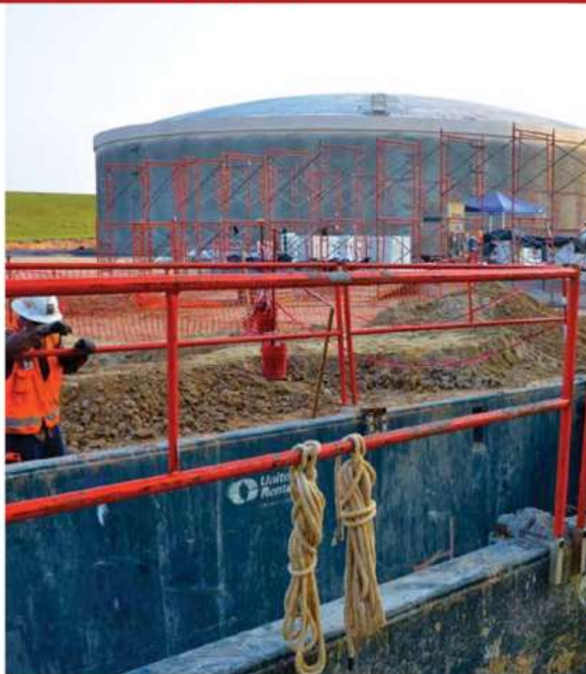
OSHA requires every excavation 5 ft or more in depth to be protected by
