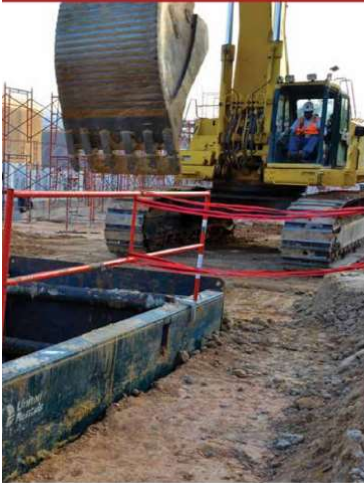
/ a trench protective system – sloping, shoring or shielding.
